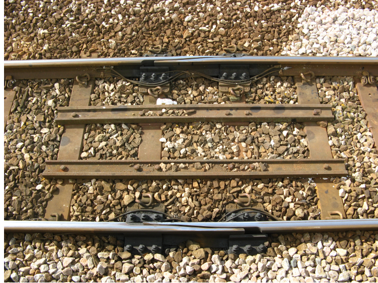
Figure 2.1: Railway track expansion joint in continuous welded rail within Hayle railway station, UK [14].
