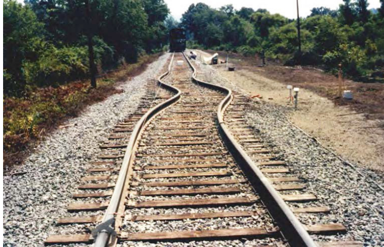
Figure 2.2: Buckling of railway track due to thermal expansion on an abnormally hot day causing [15].
